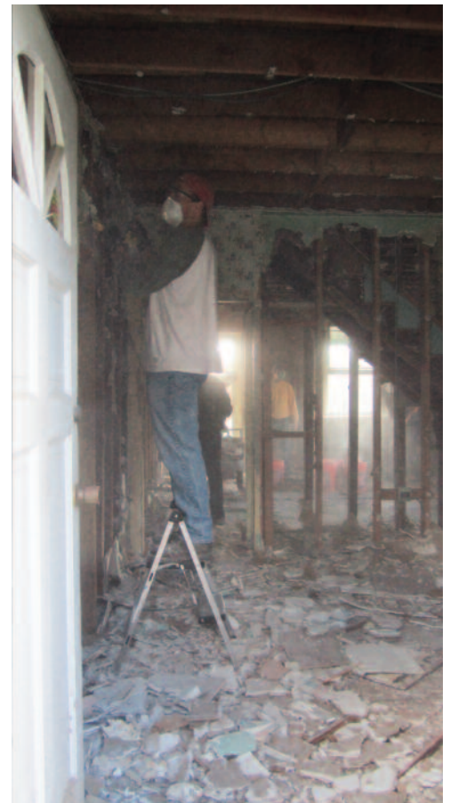
Work in progress on October 22 at 10 Folly Road.
